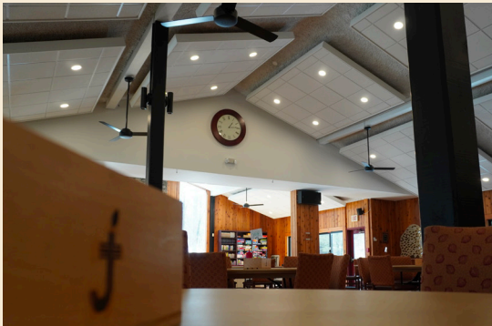
New ceiling clouds include LED lighting and fans in the main dining room as well as the conference room.
